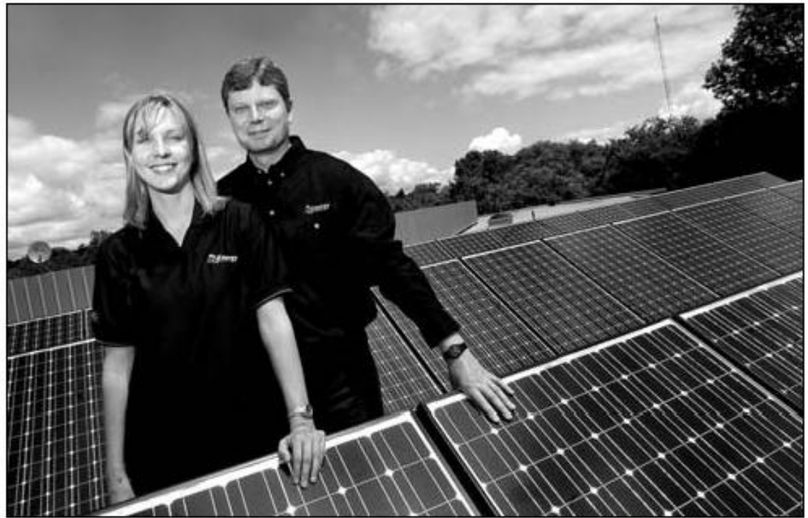
Tina McAuley and Richard Mash of FireFly Energy stand among the solar panels yesterday that have been installed on the roof of their new office building on Speedvale Avenue in Guelph.
